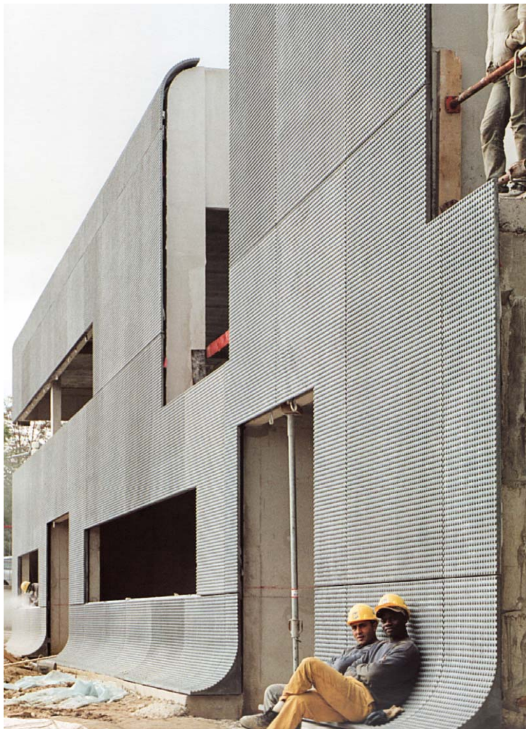
69. Cantiere, Centro Bus RATP, ECDM, Thiais
