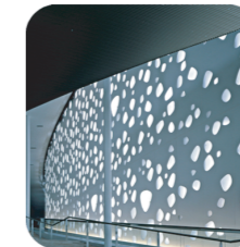
Performing Arts Center Ito, Tokyo
