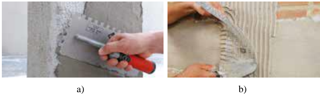
Figure 6.3 - Mortar matrices: a) Mineral Mortar (GLT); b) Natural Hydraulic Lime Mortar (GCF) [Kerakoll catalogue]
