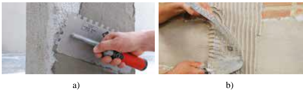
Figure 8.2 - Mortar Matrices: a) Mineral Mortar (GeoLite); b) Natural Hydraulic Lime Mortar (GeoCalce Fino) [Kerakoll catalogue]
