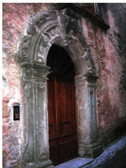
Fig.3. Building 1: "Calabria Palace", Fuscaldo (CS), XVI century
