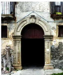
Fig.3. Building 1: "De Seta House", Intavolata (CS), XVIII century
