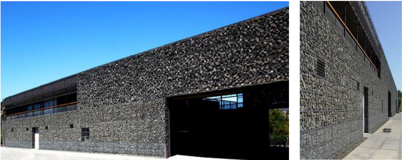
Fig. 2.9 b. Views of Dominus Winery in Yountville (California, USA), completed in 1998 and designed by Herzog & de Meron. It is characterized by gabion baskets filled with local field stone, hand stacked- to form the skin of the building which allows natural light to filter into the interior spaces, (pictures from https://www.dezeen.com/2007/09/09/dominus-winery-by-herzog-de-meuron/ ).
