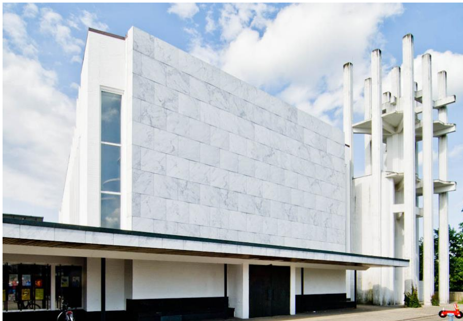
Fig. 2.7. View of Stephanuskirche in Wolfsburg (Germany), completed in 1968 and designed by Alvar Aalto. This modern religious building has a façade clad in Carrara marble, (picture from http://www.archdaily.com/372492/ad-classics-stephanuskirche-alvar-aalto ).
