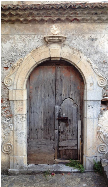
Fig.3. Building 1: "Cupido Palace", Scalea (CS)
