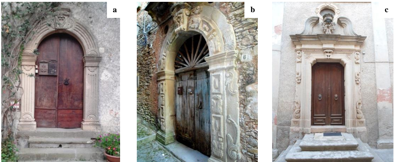
Figs. 3.46 (a, b, c). Examples of portals built with “Fuscaldo sandstone” in Fuscaldo: Carnevale Palace (a); Valenza Palace (b); Vaccari Palace (c).
