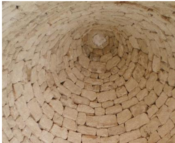
Fig. 2.3. View of “false vault” in a “Trullo” in Alberobello (Apulia, Italy), UNESCO listed in 1996, (picture from https://en.wikipedia.org/wiki/Trullo ).
