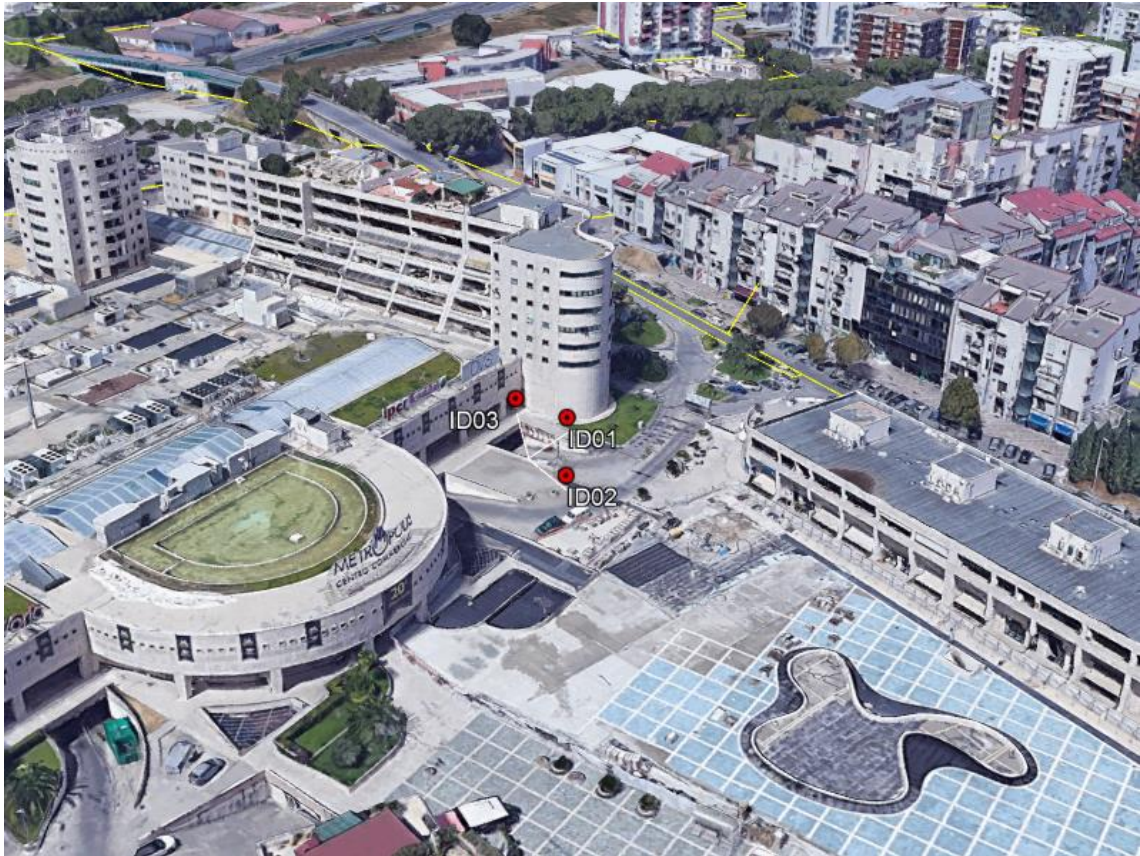
Figure 9.5.8 NB-IoT meter positioning, 3D Google terrain model.
