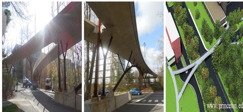
Fig. 4.60 – Streicker bridge at Princeton University campus – Princeton, NJ
