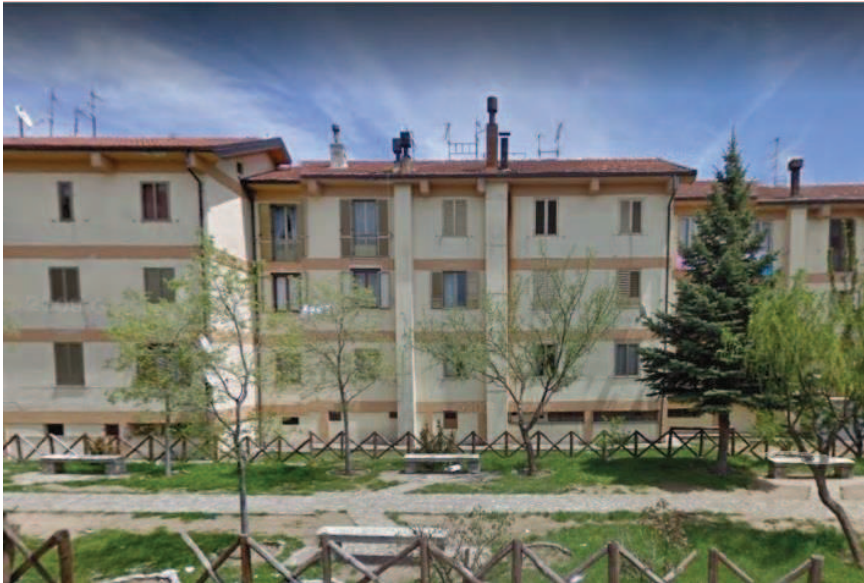
Figure 3. External view of the real reference building involved in the investigation.
