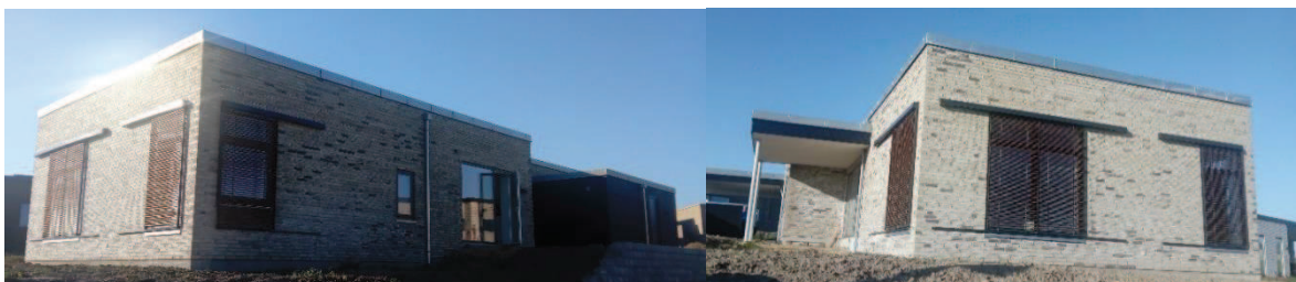
Figure 3. External views of the nZEB located in Aarhus, Denmark.
