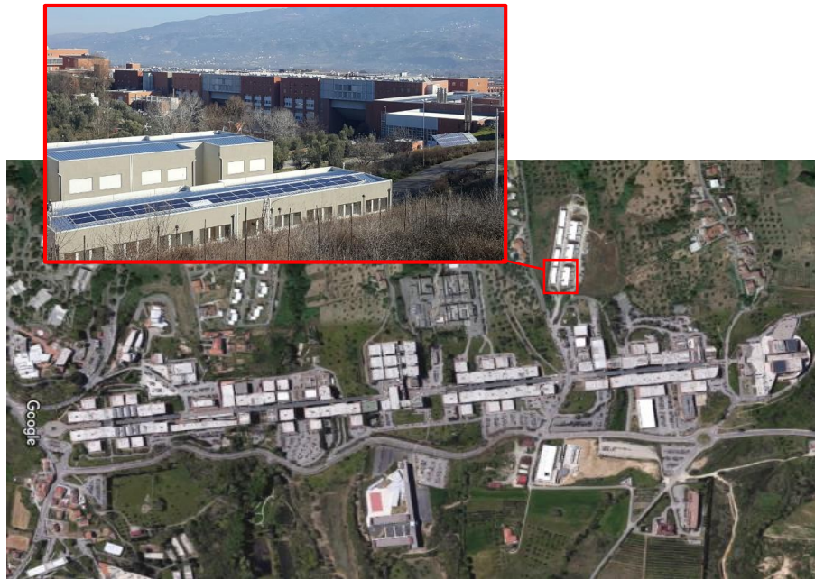
Fig. 5-4 View of the building where the system is installed
