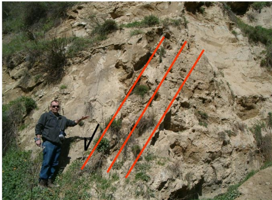
Figura 6.3: Fault zone , con faglia principale N30-70^{\circ} NO (pitch 90^{\circ} ) ed associate N35-60^{\circ} NO, N25-58^{\circ} NO, N10-50^{\circ} O.
