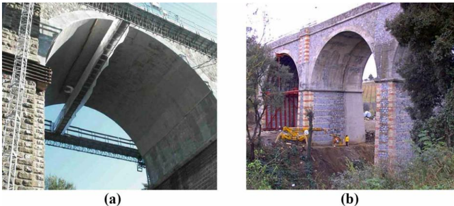
Fig. 2.12: Strengthening of railway bridge: (a) & (b) installation of the FRCM systems [54,55].
