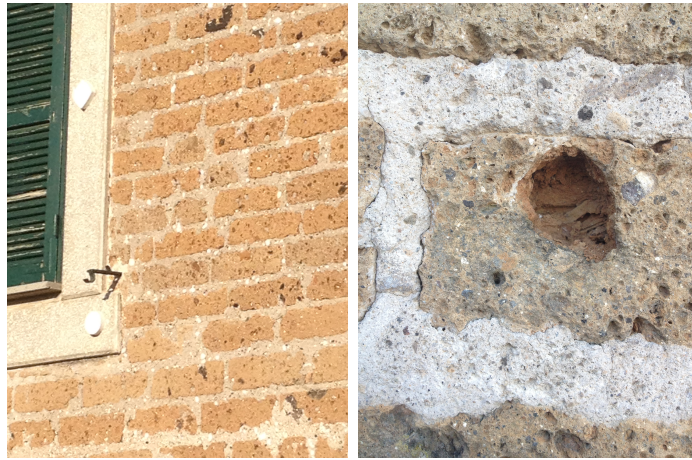
Figure 4.4: A house of Lazio Region using tuff building materials for external walling (left) and a particular of a tuff brick (right).
