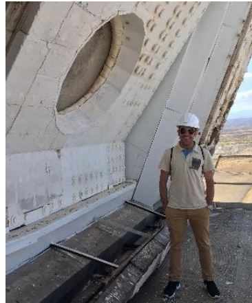
Figure 1.33: Cavity aperture on CESA-1 Tower on “Plataforma Solar de Almeria”
