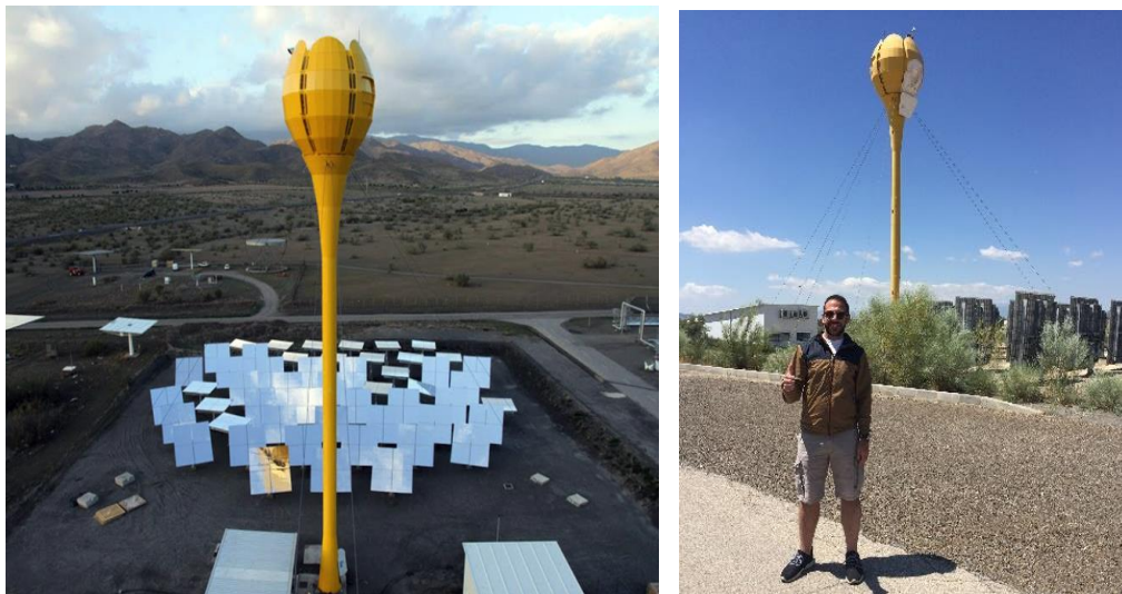
Figure 1.47: Aora Solar Plant on “Plataforma Solar de Almeria”
