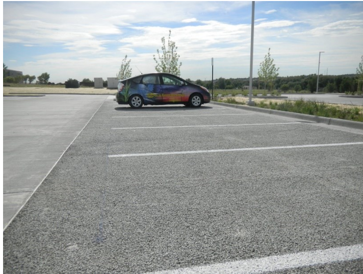
Figure 2.4 Car park constructed of porous concrete ( www.coloradohardscapes.com )
