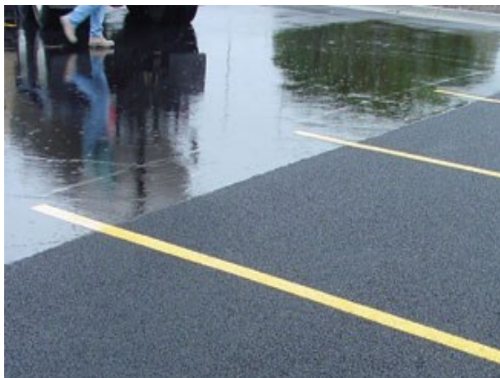
Figure 2.2 Car park constructed of Porous Asphalt ( www.wolfpaving.com )
