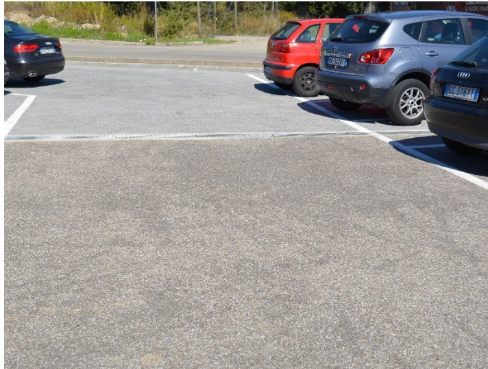
Figure 2.1 Car park constructed with PICP at Unical University
