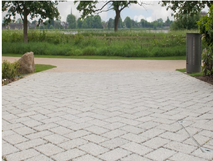
Figure 1.2 Permeable pavement ( www.marshalls.co.uk/watermanagement )
