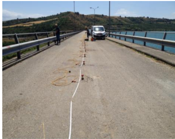
Figure 3.18: Execution of the MASW test and positions of the receivers.
