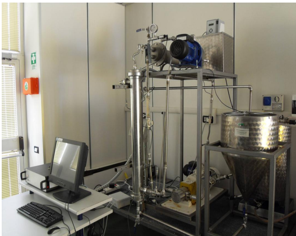
Figure 5.2 Membrane crystallization plant
