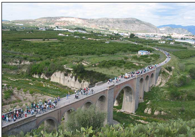
Fig. 4.15 : Puente de la Muela, Cehegin (Murcia, Spain) (fonte ceheginet.com)
