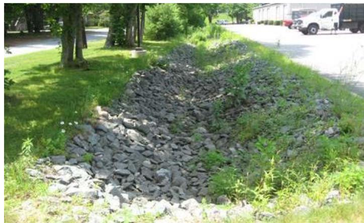
Figura 2.30: Trincea drenante presso Rhode Island, USA (<http://www.ristormwatersolutions.org>).
