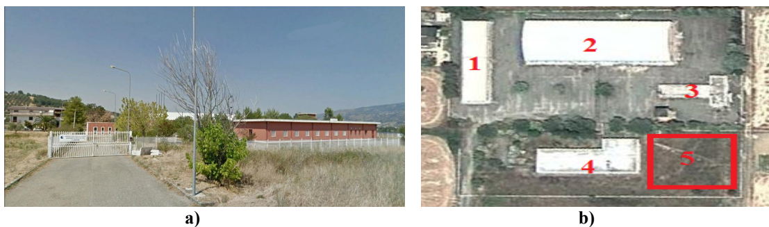
Figure 2. 22: a) Experimental well field of University of Calabria, b) 1 office 2 laboratory hydraulic models 3 warehouse 4 laboratory analysis of water and 5 field tests.
