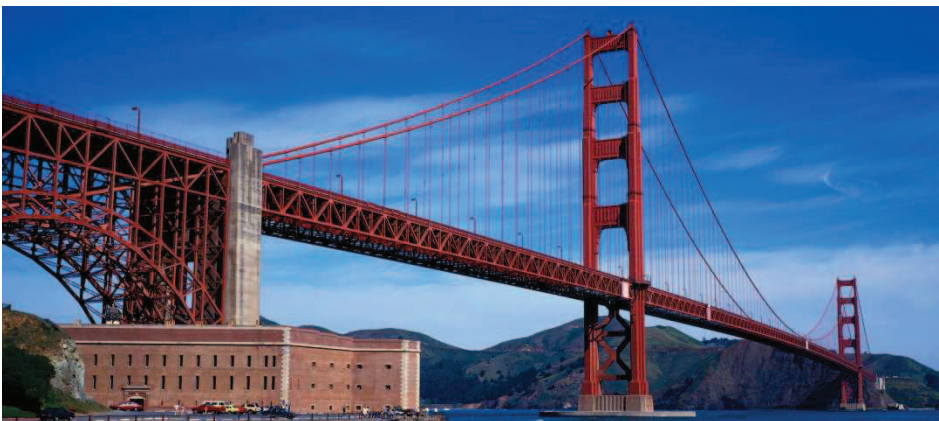
Figure 1.2 The Golden Gate Bridge
