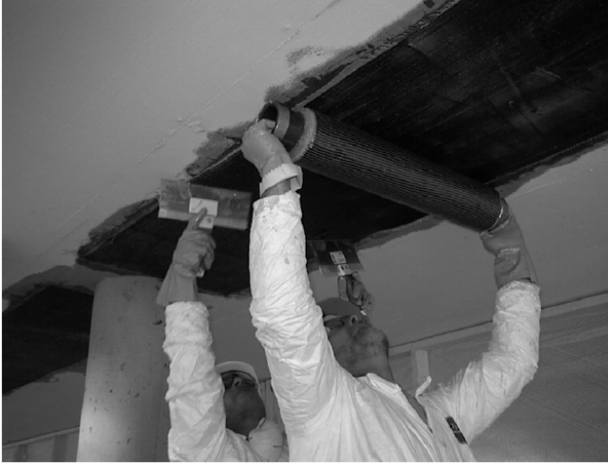
Figure 1.14: FRP sheets installation. Reprinted from [4]
