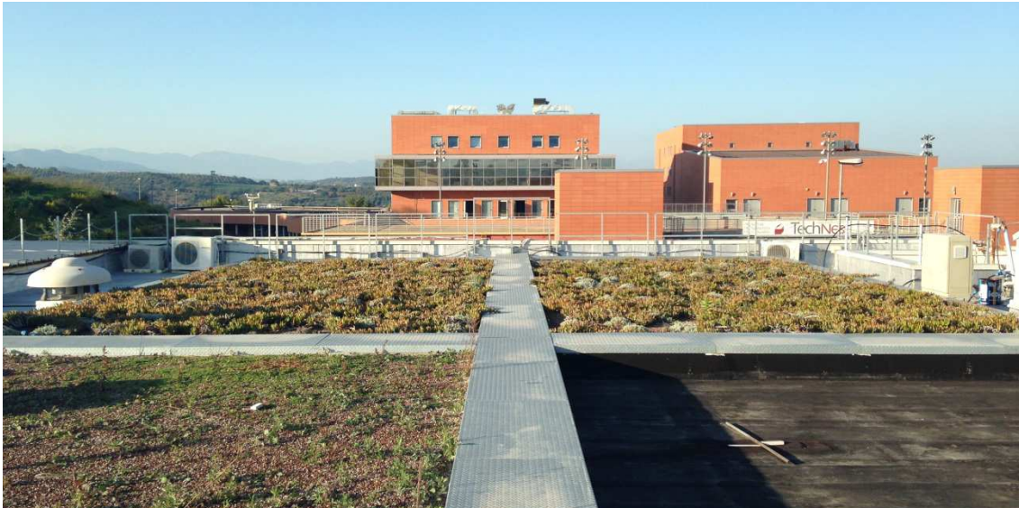
Fig. 5.2 The 4 compartments of the Unical Experimental site.
