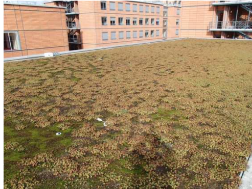
Figure 4.4. View of the Lyon Congress Centre green roof (photo LGCIE-DEEP).
