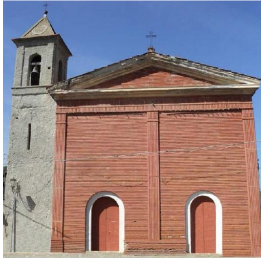
Figure 4.1: Present elevation of the Santa Maria dei Longobardi church, in San Marco Argentano.
