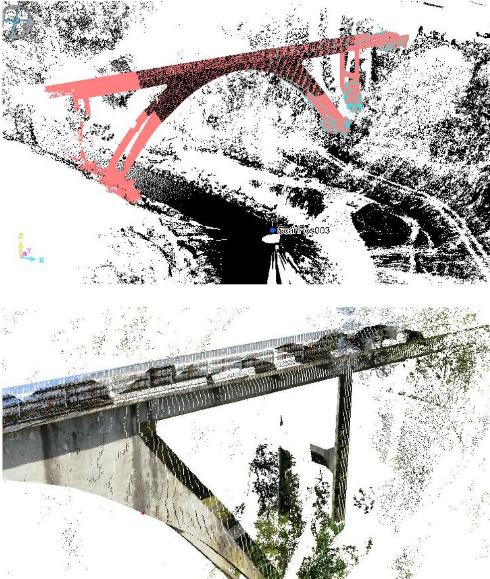
Figure 5.6 Union of scans and detail of a colored point cloud.
