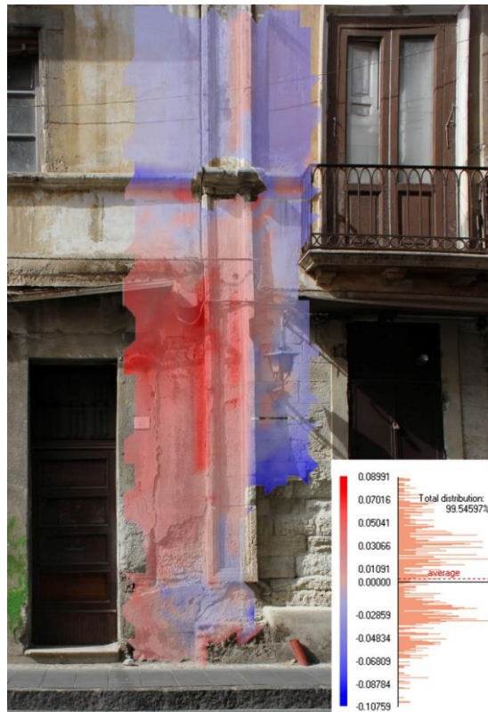
Figure 2.4: The deviations with respect to the average vertical plane are highlighted in colors: in red the positive protrusions.
