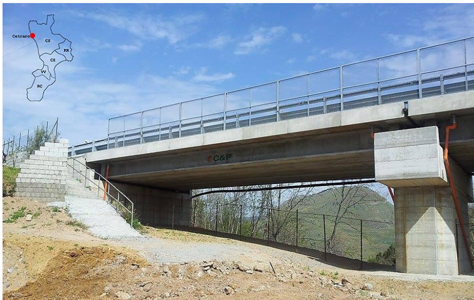
Figure 5.2 The Arenazza bridge.
