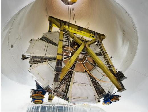
**Figure 3.1:** Picture showing the lowering of the ATLAS Small Wheel. On the front side are visible the 8 MDT chambers placed on a ring structure, while in the inner part of the ring the 8 TGC chambers are partially visible. Moreover 8 CSC chambers are installed in the Small Wheel but not visible.
