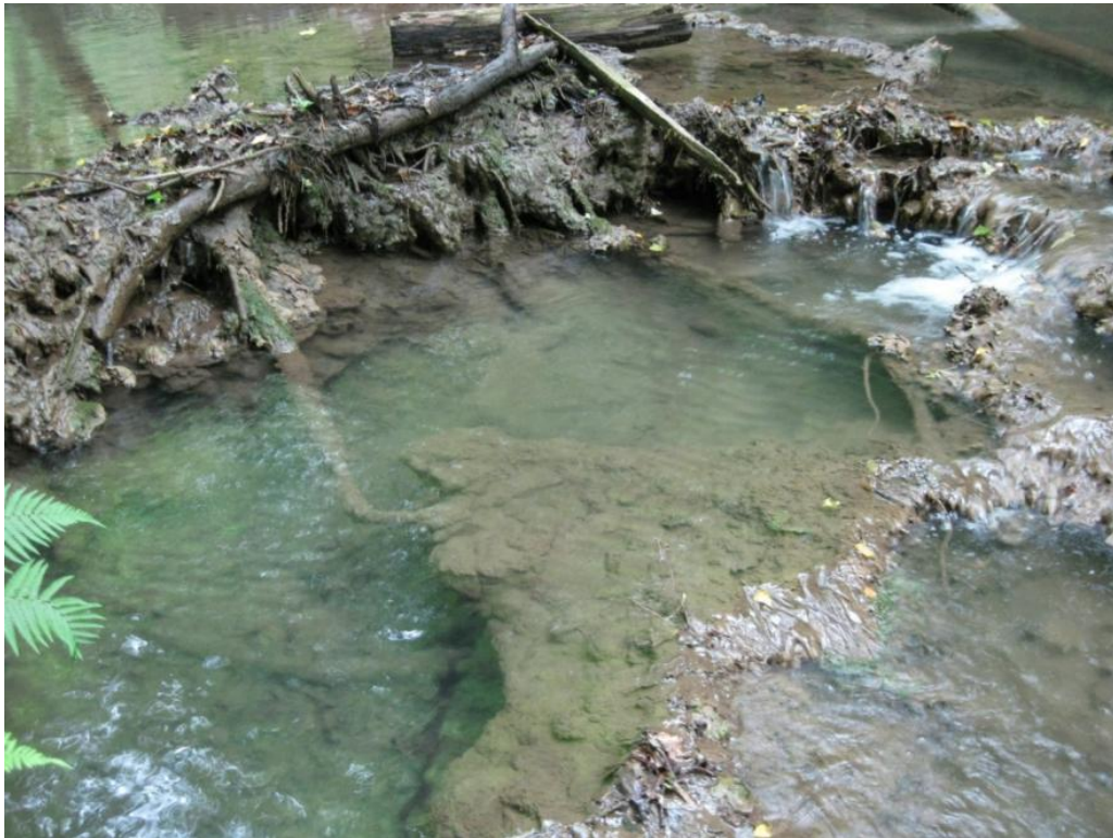
Fig. 4.11. Barrage up-stream wall developed pool behind the barrage.
