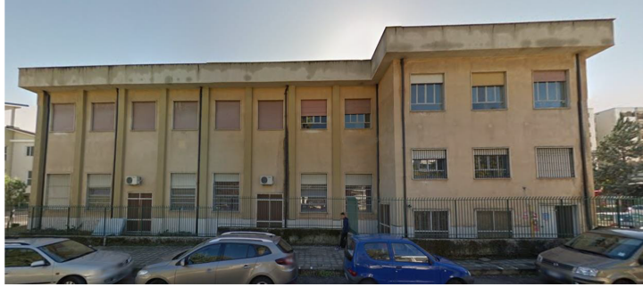
Figure 5.2: Auditorium of the Industrial Technical Institute A. Monaco
