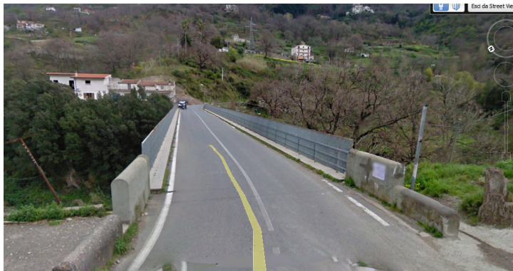
Figure 4.29: Caprovini Bridge: view of the top road
