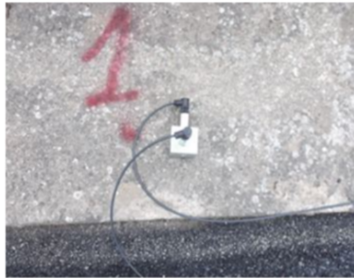
Figure 4.10: No.2 monoaxial accelerometers combined on the basis for biaxial readings
