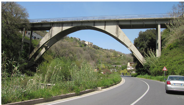
Figure 4.30: Caprovini Bridge: view from the valley to the mountain
