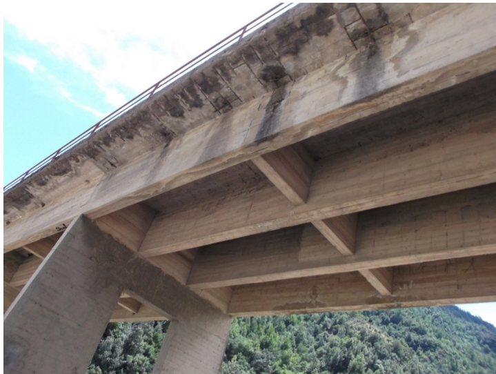
Figure 4.5: Fiume Trionto Bridge: bottom view
