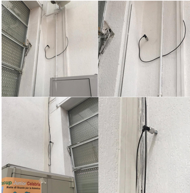
Figure 5.17: Position of accelerometers (no.1, no.2): ground floor
