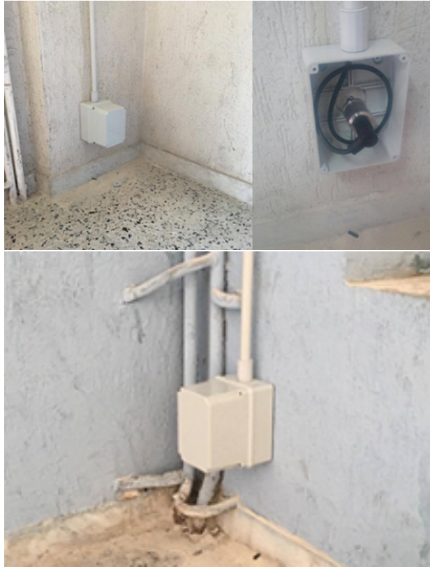
Figure 5.18: Position of accelerometers (no.3, no.4): ground floor
