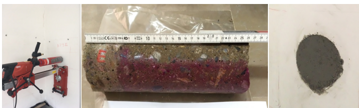
Figure 5.10: Core test:HILTI DD150-U diamond drilling systems, Measurement of hardened concrete carbonation depth, Hole sealing material
