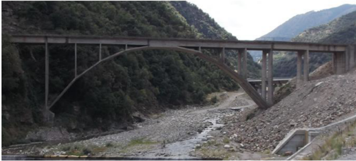
Figure 4.1: Fiume Trionto Bridge: view from downstream towards upstream.
