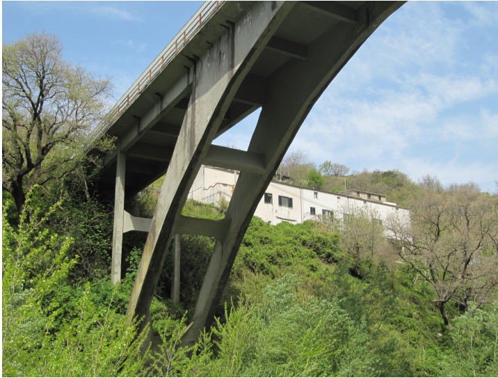
Figure 4.31: Caprovini Bridge: view from below
