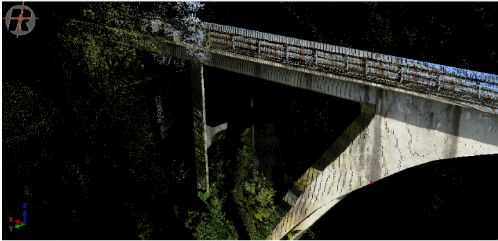
Figure 4.34: Caprovini Bridge: detail of scanning the support of the crutch parabolic reinforced concrete
