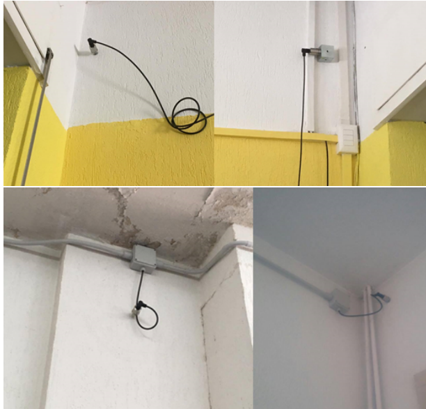
Figure 5.19: Position of accelerometers (no.5, no.6, no.7, no.8)
