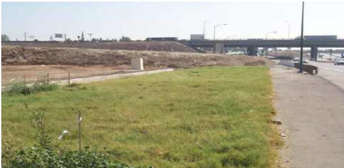
Fig. 3. 12 - Vegetated filter strips (CASQA, 2003).
