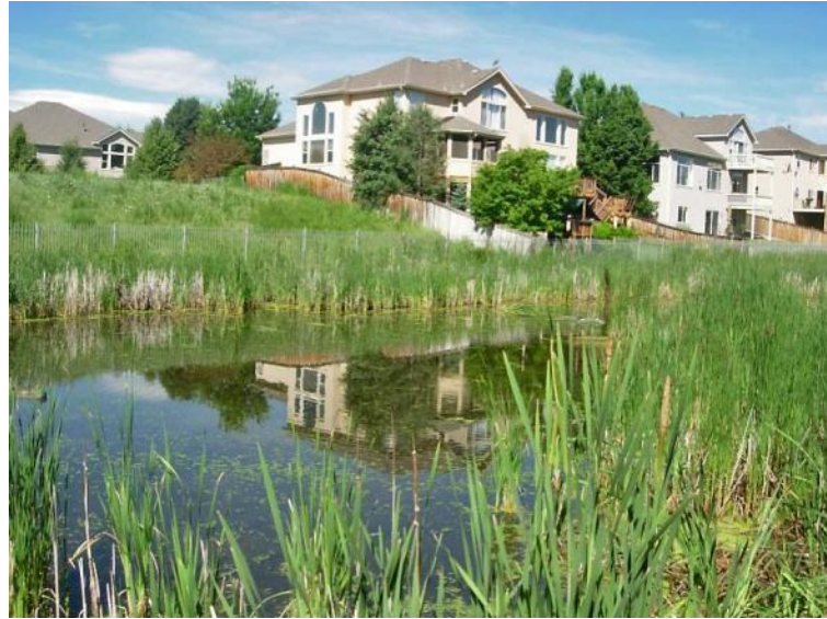
Fig. 3. 21 – A constructed wetland pond, located downstream of an extended detention basin (USDCM, 2010).
