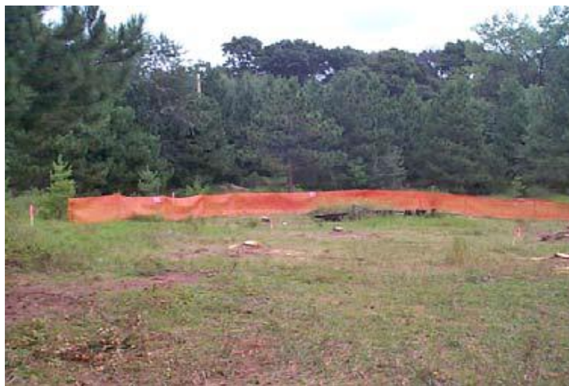
Fig. 3. 3 - Minimizing disturbance of soil to protect wooded area Source: City of Andover, Minnesota.
