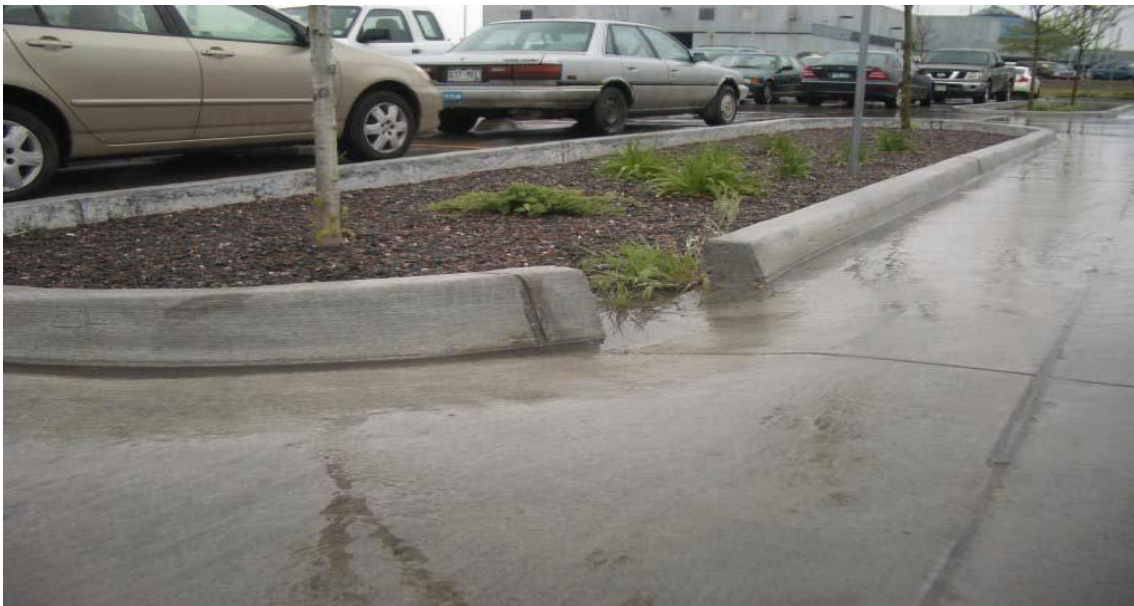
Fig. 3. 13 - Bioretention area or ‘rain garden’ installed in a car park (USDCM, 2010).
