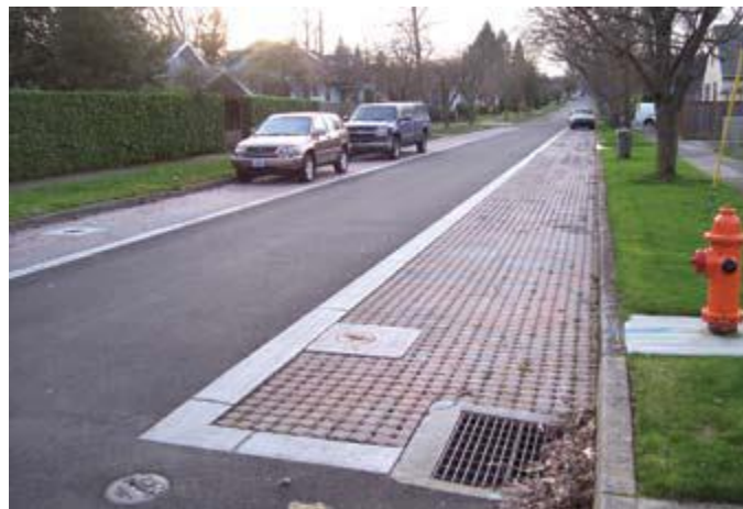
Fig. 3. 8 - Use of permeable pavers for roadway shoulders.
