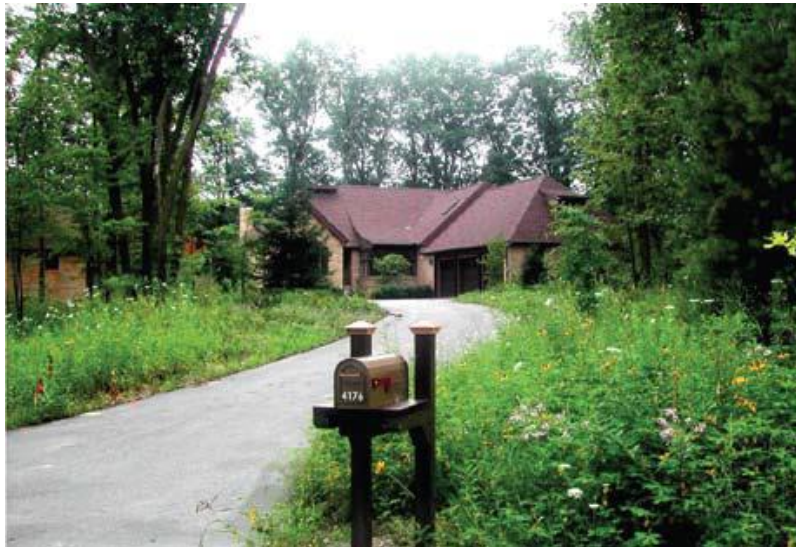
Fig. 3. 4 - Minimizing disturbance to existing trees during residential construction. Source: Insite Design Studio, Inc.
